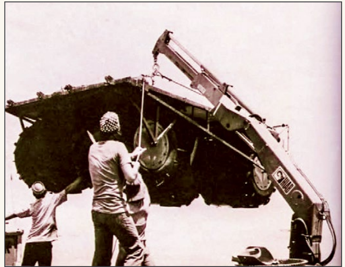
Figure 6: The Seiga being lifted onto the helideck.
