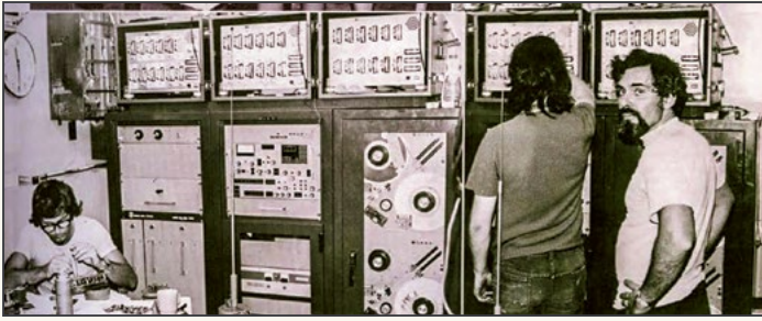
Figure 2: Party 101 instrument technicians at work in the recording room of the Western Beach. The lower rack contains the DDS 888 recording system with IBM 3480 tape drives. The Telseis instruments are in the upper rack.
